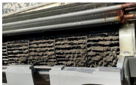
Presence of mould, fungus and mildew in the air conditioning systems
