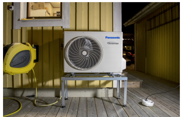
4. Mount the crossbars and adjust to your heat pump.
