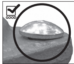
Oval Neck of Bolt Seated Properly
