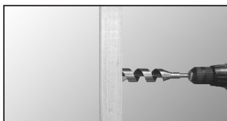
Bor 32mm hull i stender.
