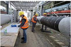
Thermal-acoustic insulation of installations at the new gas processing plant in Etzel (Germany); reliable protection against corrosion under insulation (CUI)
