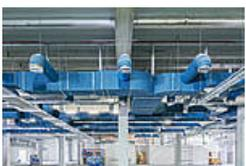
Premiere on the building site: even before it was officially launched, the new enhanced ArmaFlex Ultima had been installed in the new Labesfal - Fresenius Kabi plant. To prevent the pharmaceutical products manufactured here being contaminated, the construction materials have to meet the stringent requirements for cleanroom technology.
