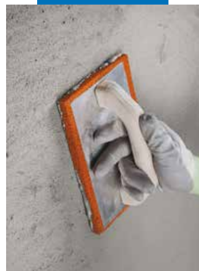
Tamping Planitop Smooth & Repair
