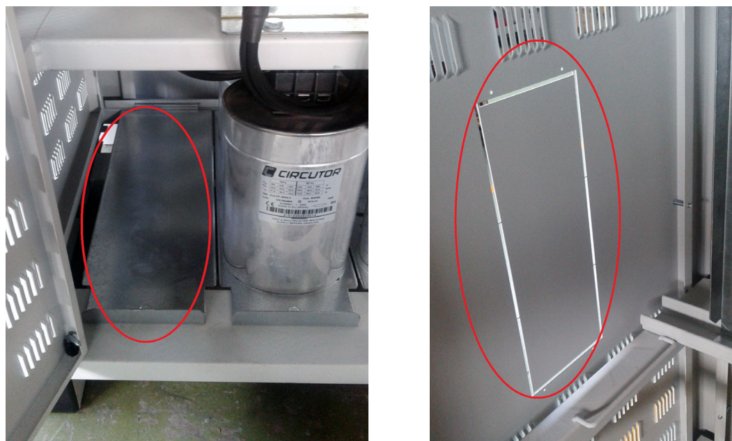
Figure 6: Cable entry points of the OPTIM FRE models.
