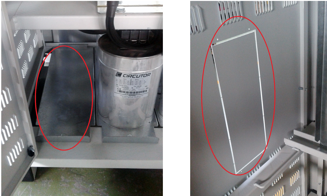
Figure 5: Cable entry points of the OPTIM FR P&P models.
