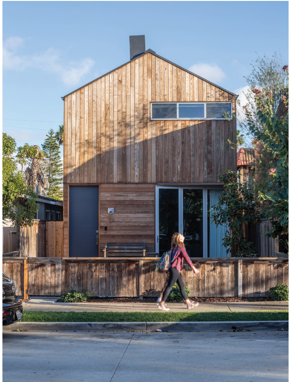
Benchmark by Thermory Thermo-ash cladding. Hidden installation with PaCS Clad (powered by Grad). Private house in USA. Designed by DIG:A
