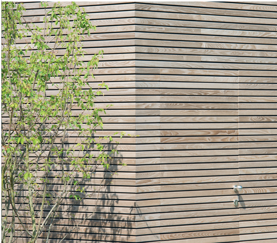
Cut the boards to a 45-degree angle.
