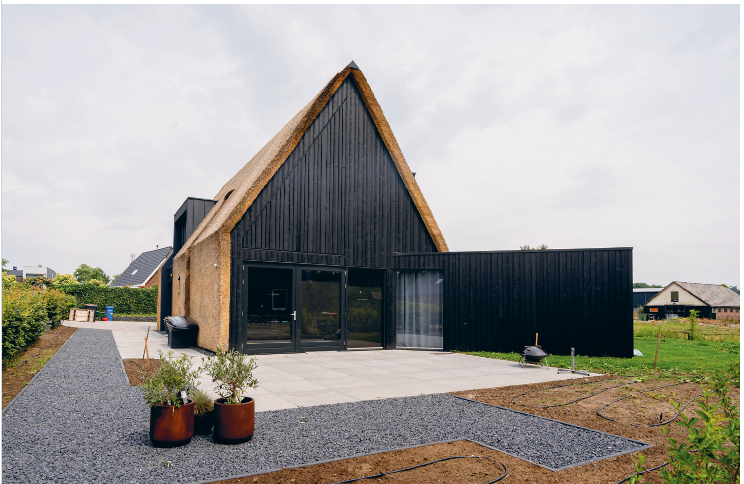
Vivid by Thermory thermo-spruce cladding (D4 / Channelsiding), color Black. Private house in Netherlands. Distribution & Photo by InterFaca
