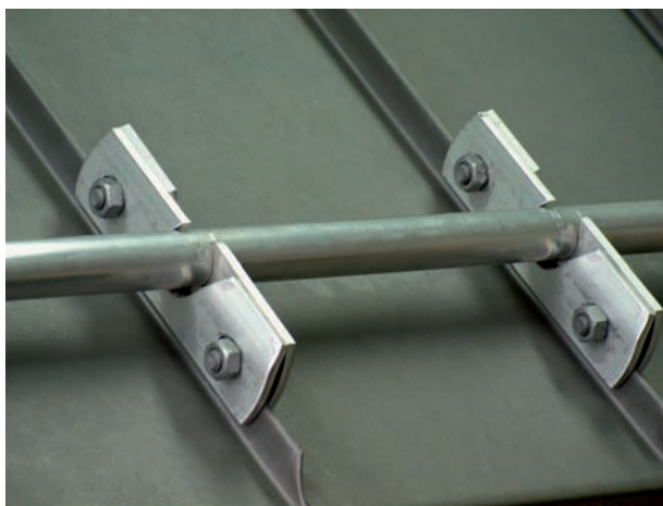
Drawing 8 The way of safety accessories fastening to the seam
